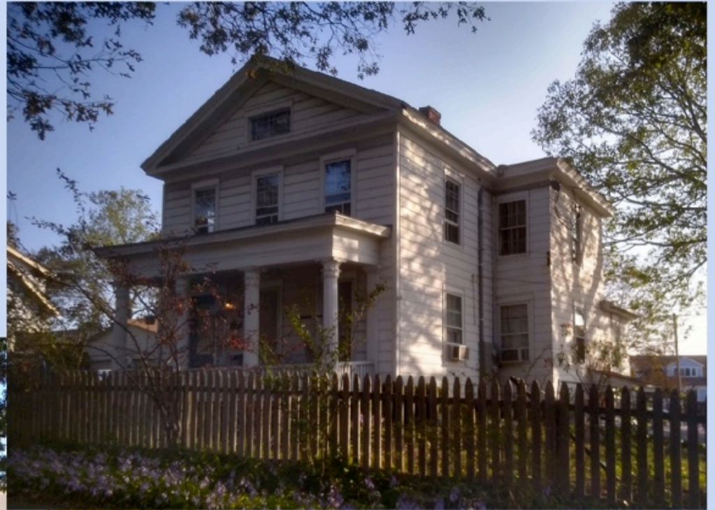
WEST View from Howard Avenue
