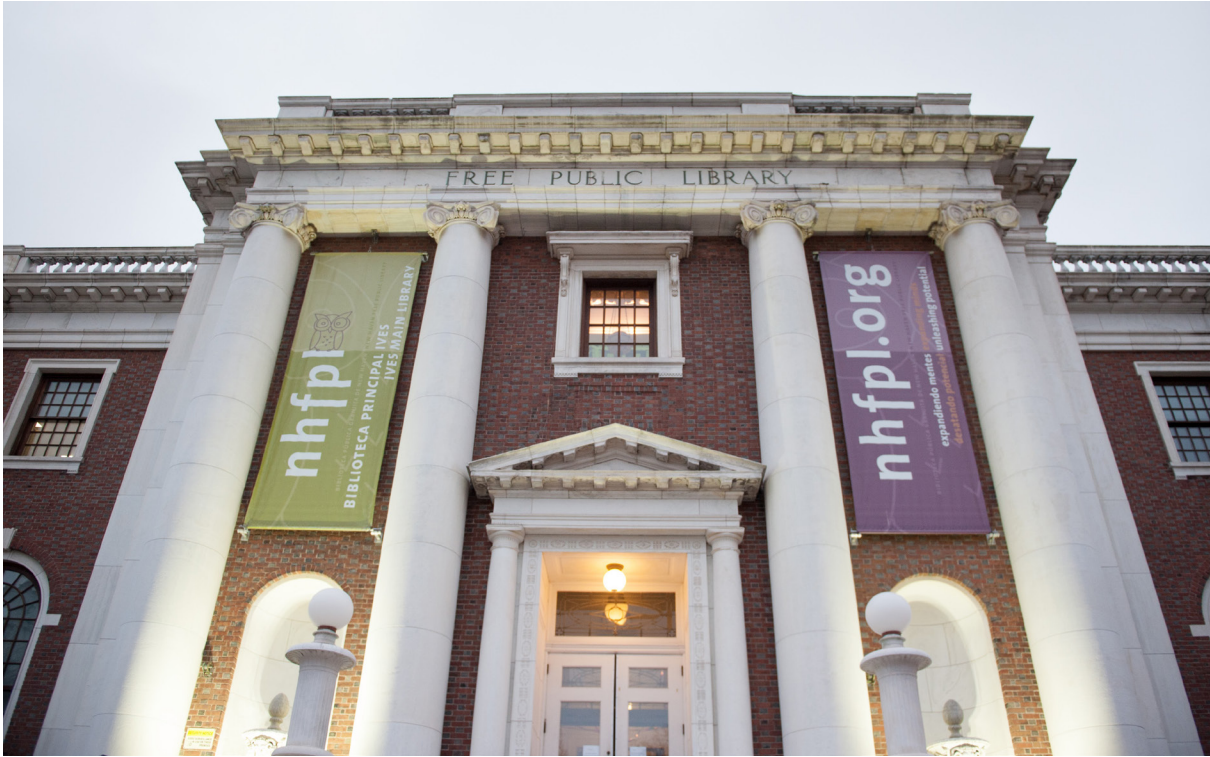
Ives Main Library, a landmark of the historic New Haven Green.
