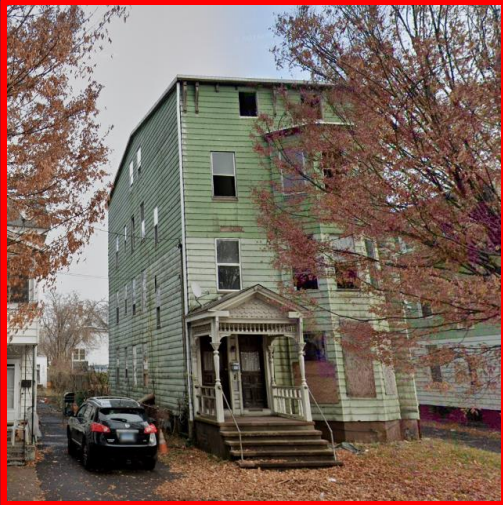
379 Ferry St Vacant home
