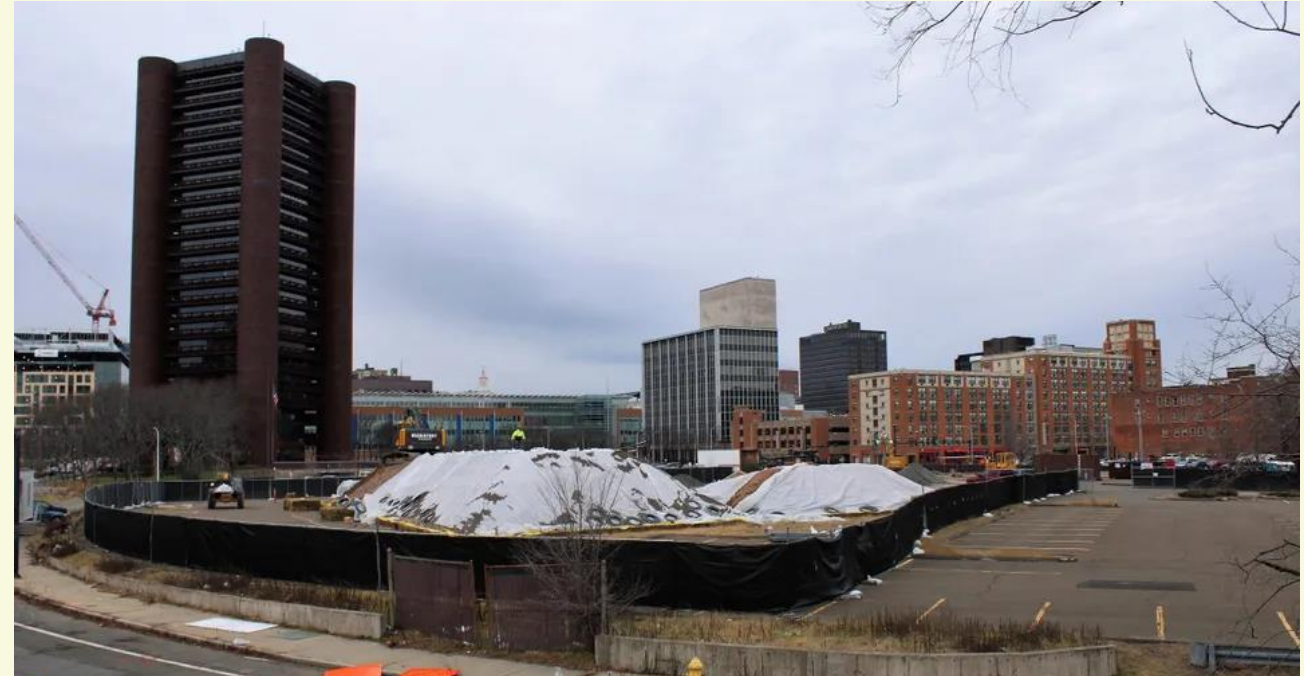
The former Coliseum site, where Phase 1A is now under construction.
