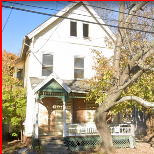
287 Division St Vacant home
