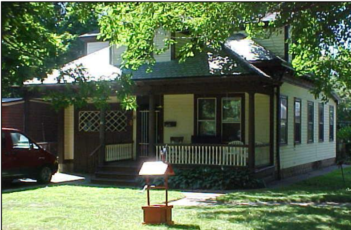
A roof replacement at 46 Sixth Street (left) in the Quinnipiac Local Historic District was reviewed and granted a Certificate of Appropriateness by the HDC at its September 2015 meeting.
