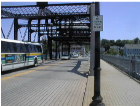
Looking east across the Grand Avenue Bridge over the Quinnipiac River.
