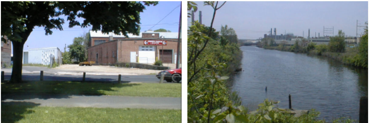
(left) Chapel Street just east of its bridge over the Mill River, where Criscuolo Park (foreground) meets Providence & Worcester Railroad right-of-way (background) (right) Looking south from the former Providence & Worcester Railroad Bridge over the Mill River
