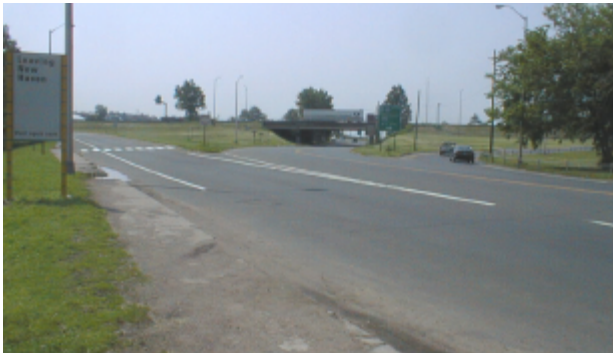
From Ella T. Grasso Boulevard looking south towards I-95. Though not visible in this photograph, Kimberly Field is to the left.
