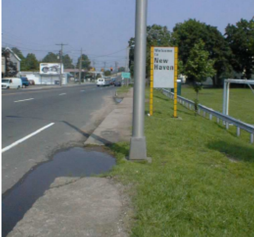
From Ella T. Grasso Boulevard looking north. Kimberly Field is visible to the right. Though the sign may welcome travelers to New Haven, pedestrian facilities along the Boulevard are un-welcoming.
