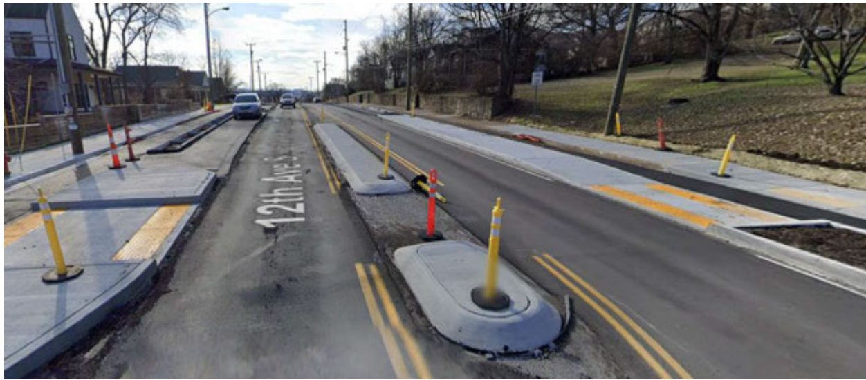
Figure 4.18 Pedestrian Refuge Island – Nashville, TN
