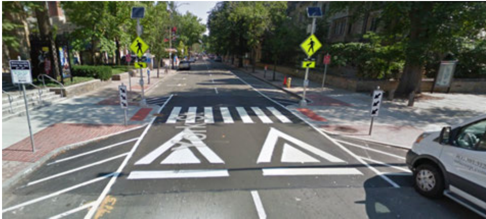
Figure 2.9 Mid-Block Raised Crosswalk on York Street
