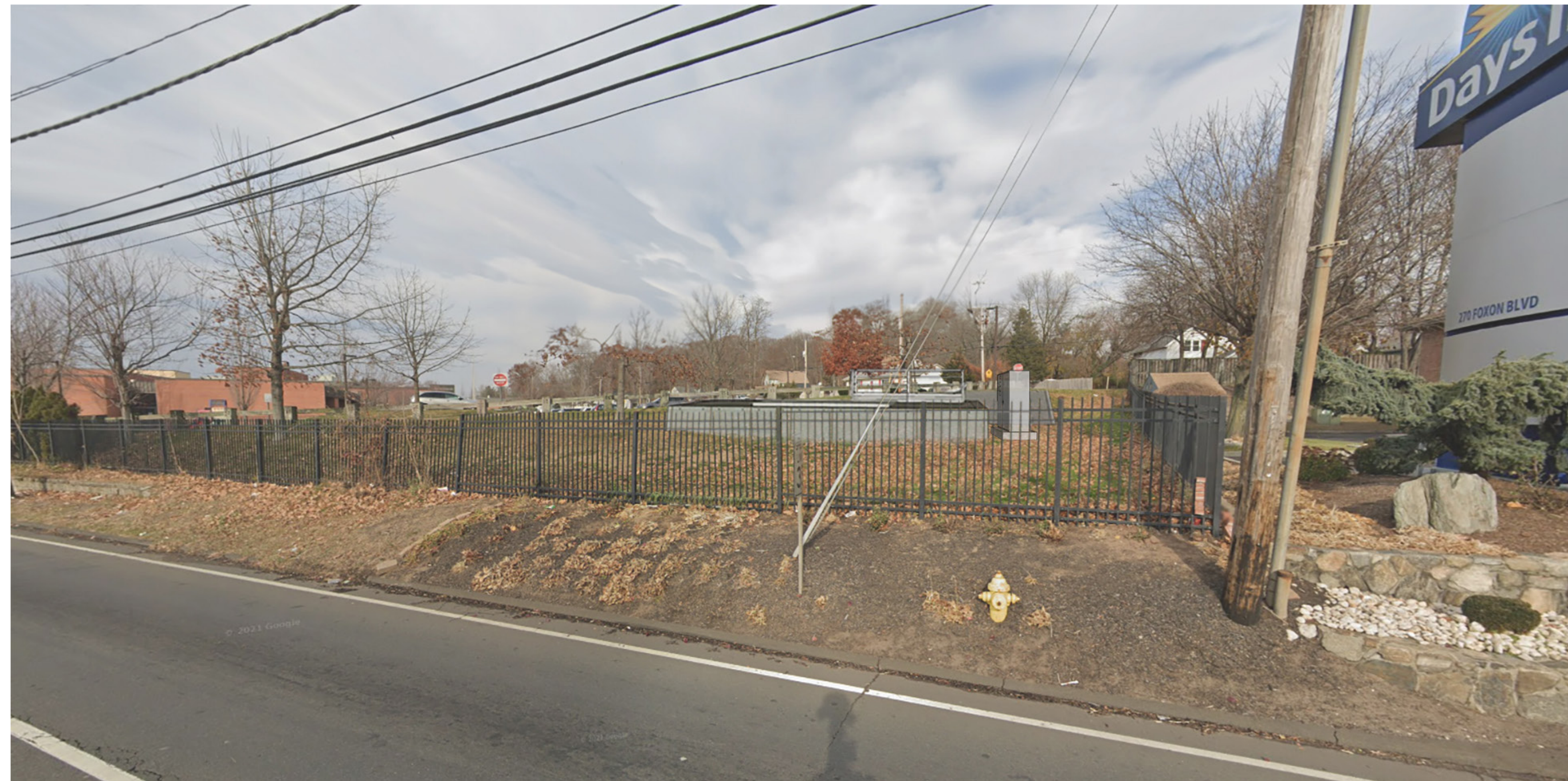
VIEW 2 - FROM RTE. 80 LOOKING NORTH
