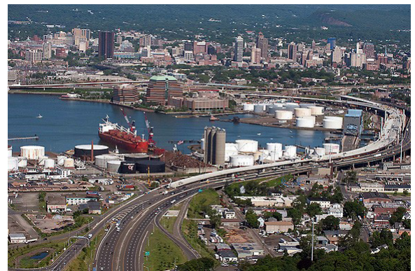
View of New Haven Port area.
