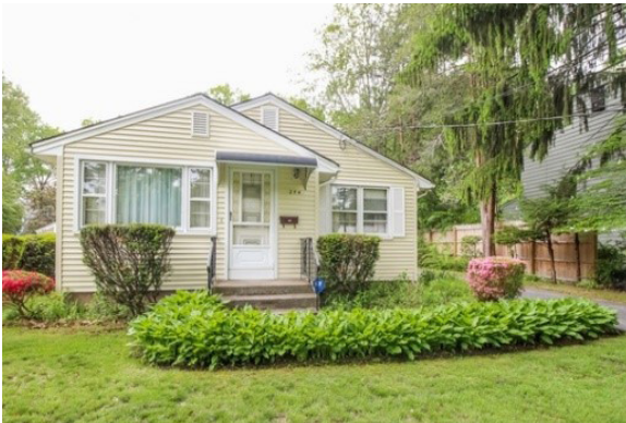
Example of a low-density residential property located on Oliver Road.
