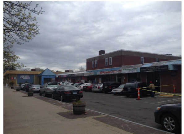
Existing view of Dixwell Plaza—a neighborhood-based commercial corridor in Dixwell neighborhood.
