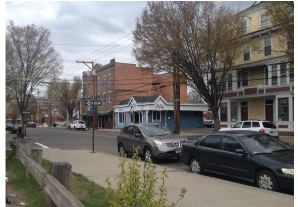
Existing view of Grand Avenue—a neighborhood-based commercial corridor in Fair Haven neighborhood.
