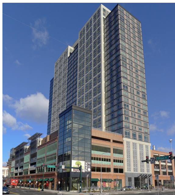
Example of Downtown residential mixed-use building on 360 State Street.
