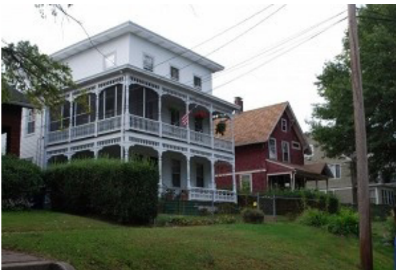
Distinctive single-family and two-/three-family houses from the mid- to late-19 th century enhance the historic character of City Point neighborhood.
