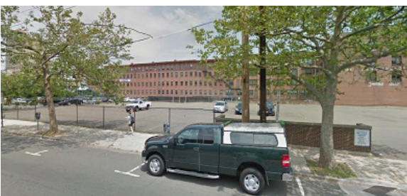
Strauss Adler Building site on Olive Street
