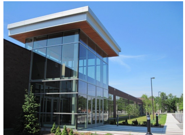
The newly built 245,000 sf office center on the historic Winchester Repeating Arms gun factory site at Science Park in Newhallville neighborhood. This building is now home to Yale's administrative offices, a print shop, and other offices
