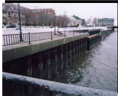
Existing bulkheads at Quinnipiac River Park
