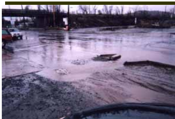
Existing stormwater runoff and collection along Middletown Avenue
