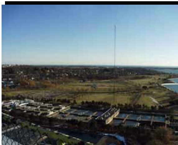
View of East Shore Park
