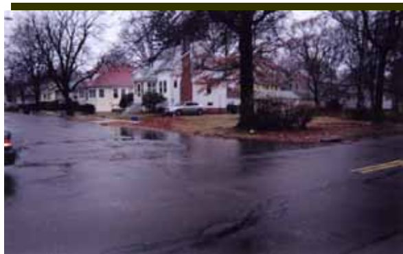
Area of poor drainage in Morris Cove neighborhood
