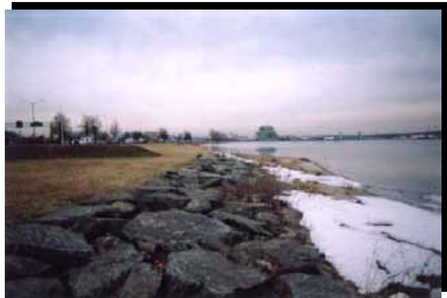
Existing erosion controls at Long Wharf Park
