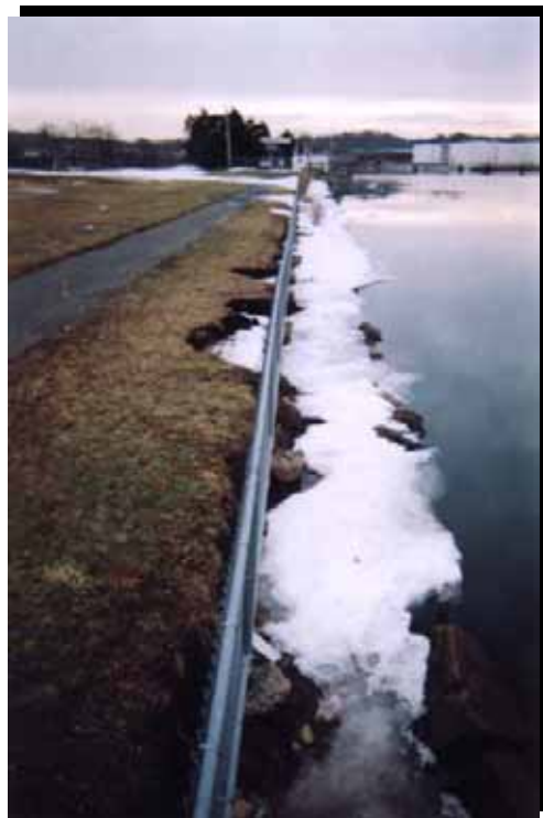
Shoreline erosion at Criscuolo Park
