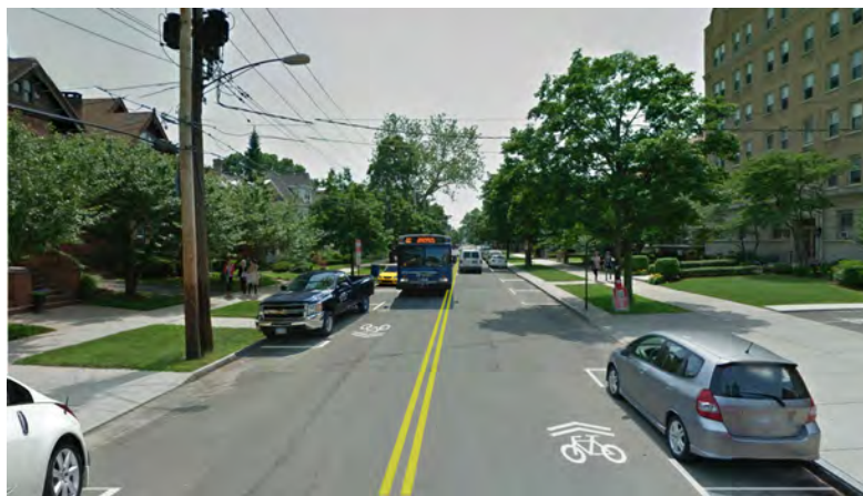
Dwight Street proposed travel lanes with sharrow and parking lanes
