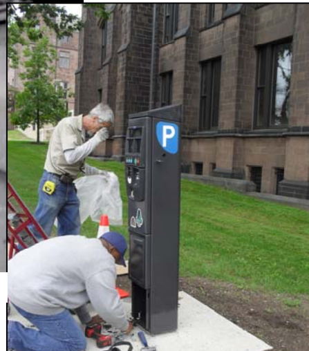
New Parking Meter Pay Station Installed on Prospect Street
