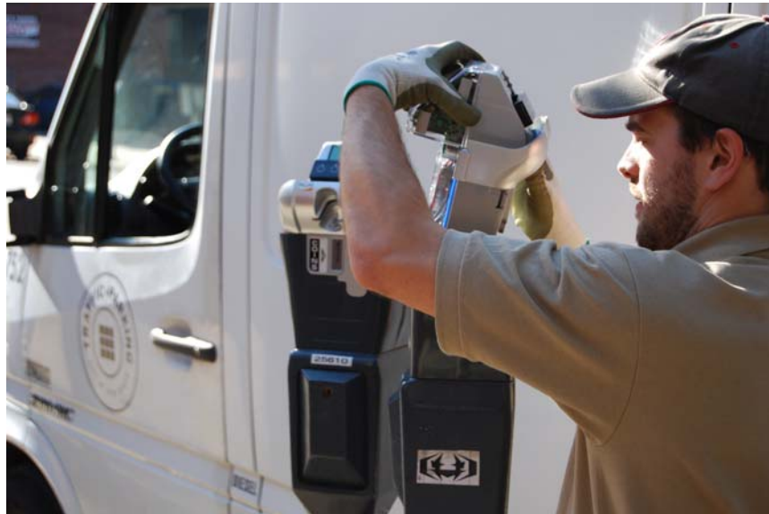
Meter Crew Installing New Credit Card Accepting Parking Meters
