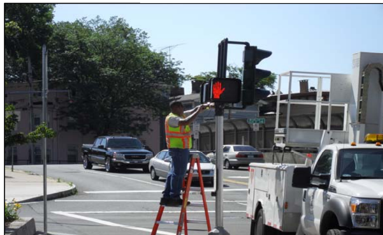
Work Performed by Signal Crew to Replace the Pedestal
