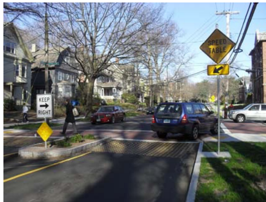
New Speed Table Installed on Edwards and Livingston
