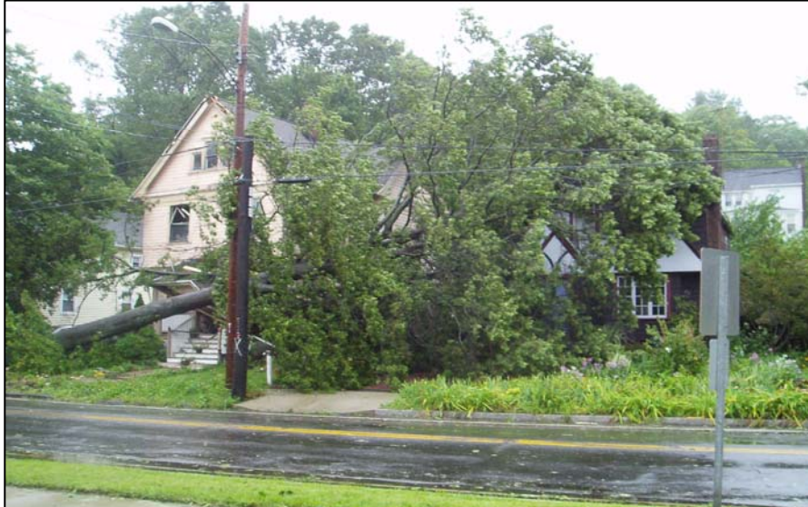
Houses Damaged on Forest Road
