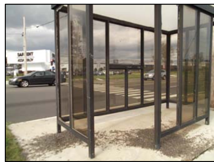
Result of High Winds Along New Haven Harbor-Uprooted a Sign and Blew Out Glass Panels of a Bus Shelter
