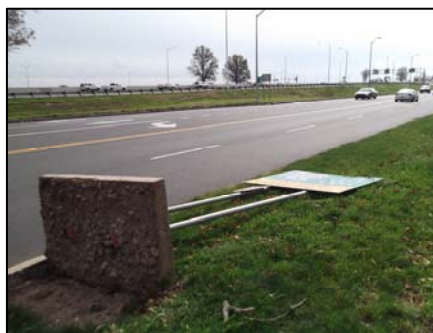
Result of High Winds Along New Haven Harbor-Uprooted a Sign and Blew Out Glass Panels of a Bus Shelter
