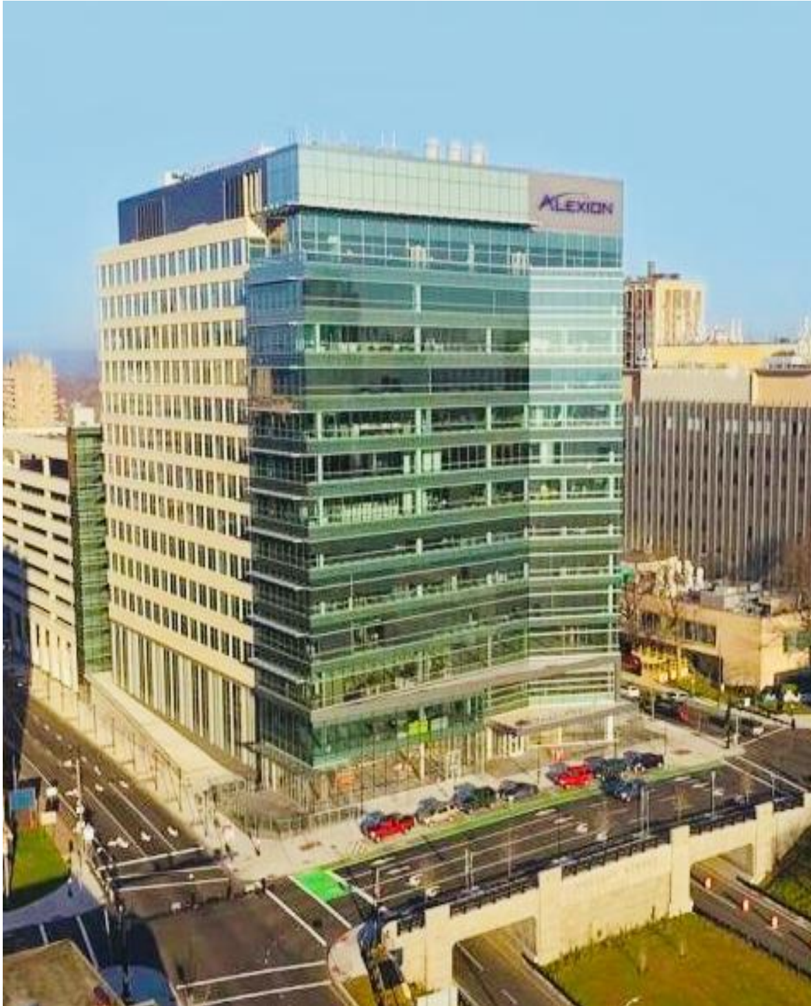
100 College Street | Construction Made Possible by Phase I of the City's Downtown Crossing infrastructure initiative.
