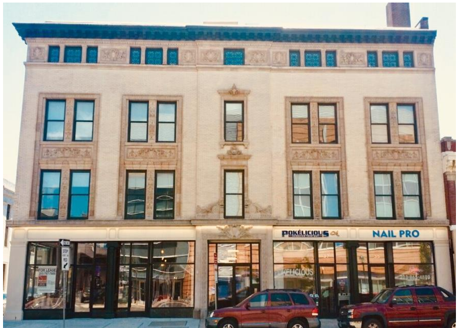
35-39 Church Street | Received a Façade Improvement Grant to restore a historic façade, create two ground-floor retail spaces, and convert the upper floors into apartments.
