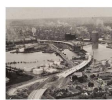
HARBOR DEVELOPMENT Construction of "G" Bridge, 1958.
