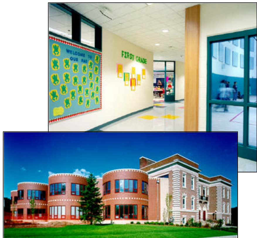
Figure 9.3: Additions and renovations to Edgewood School.
