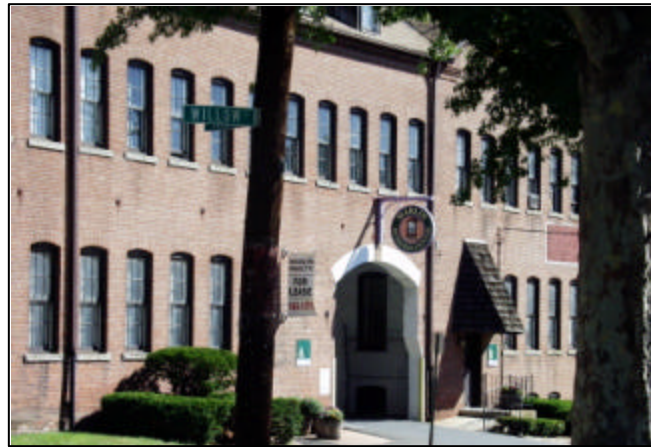
Figure 5.1: Adaptive reuse of the former Marlin Firearms, Willow Street
