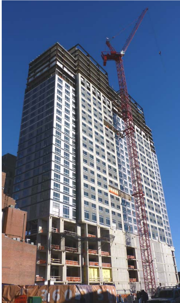
360 State Street Tower Under Construction
