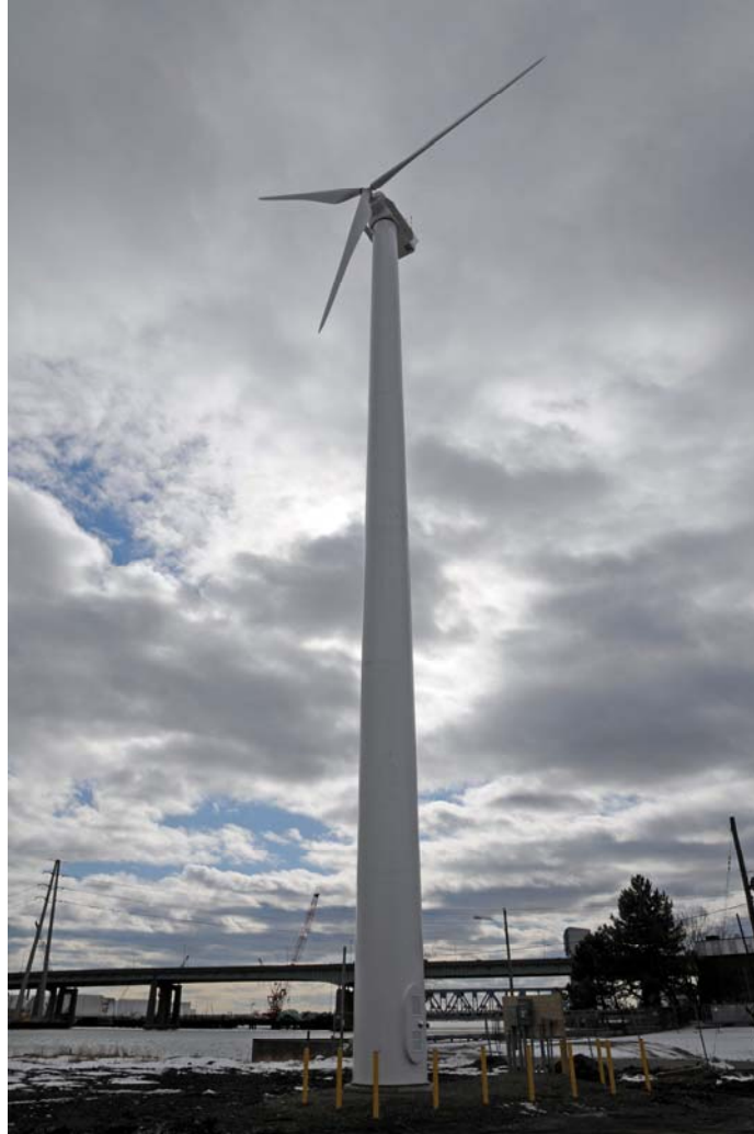
Phoenix Press Wind Turbine
