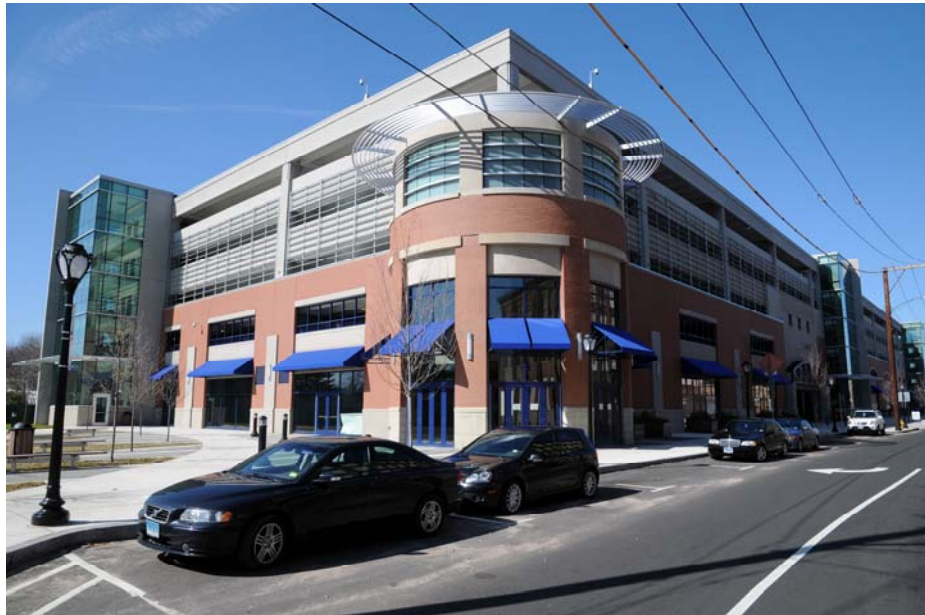
Science Park Parking Garage with Street Level Retail
