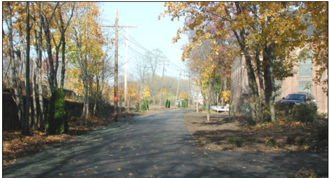
FCL Phase I – under construction
