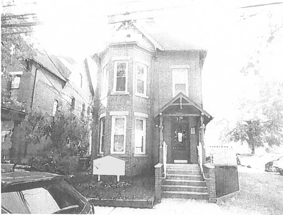
FRONT VIEW OF SUBJECT FACING SOUTHERLY
